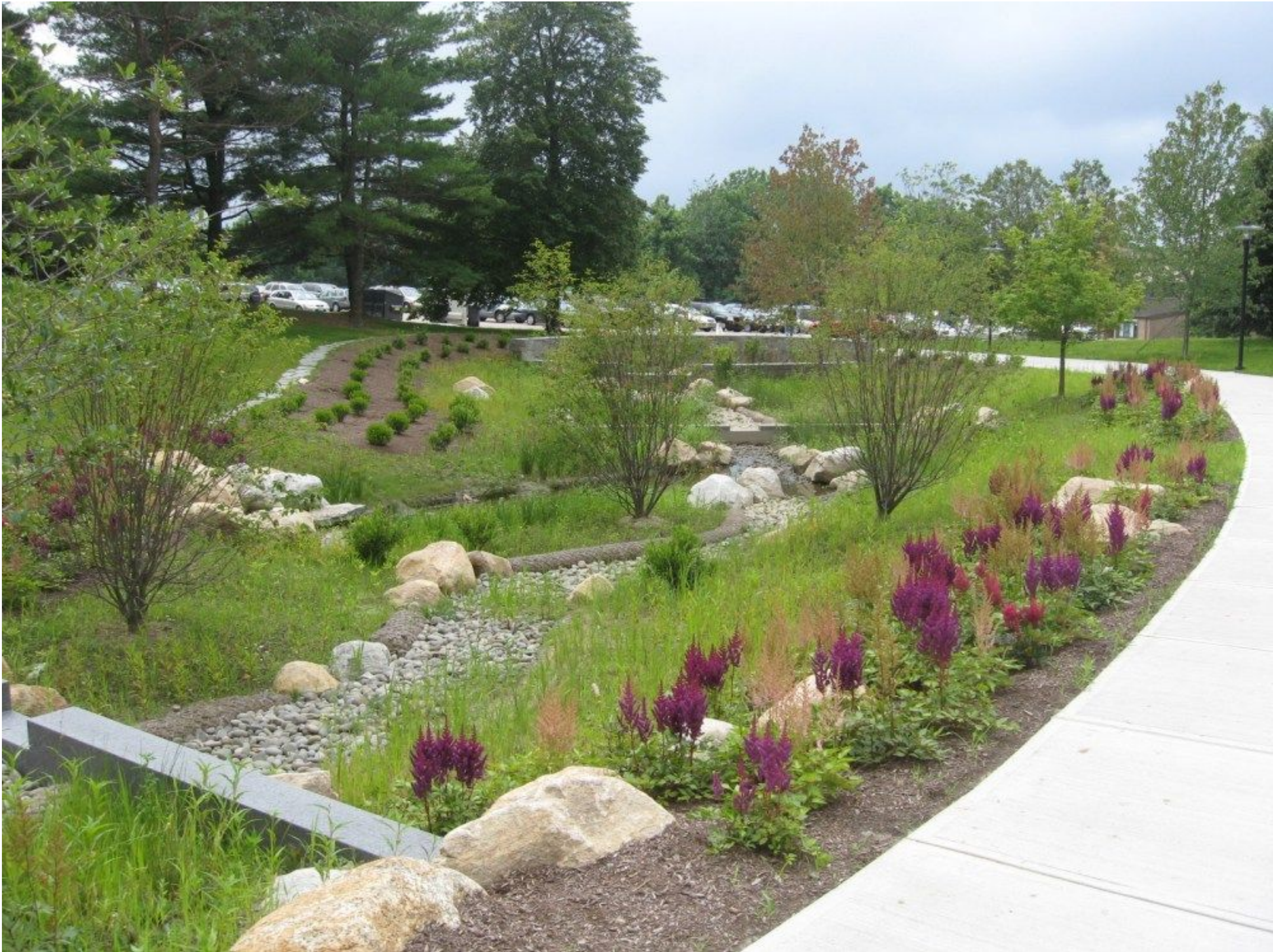
Bioretention basins use native plants and materials to slow and infiltrate stormwater runoff.
