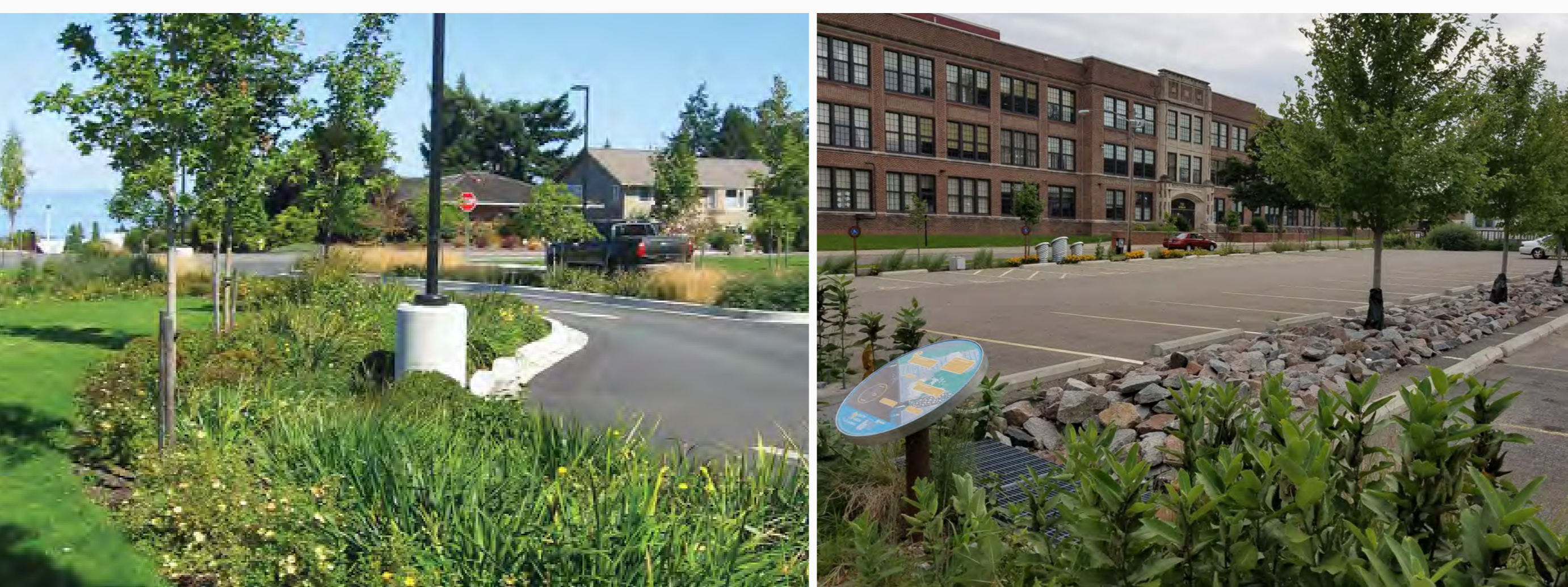
Examples of stormwater features such as planted swales and retention basins integrated in development
