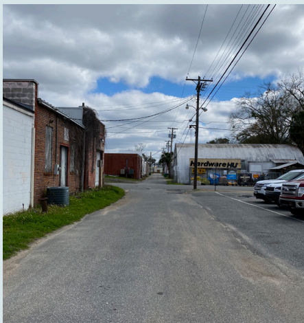
Existing conditions at South Alley Street and City Hall parking lot (proposed location for green alley and City Park)
